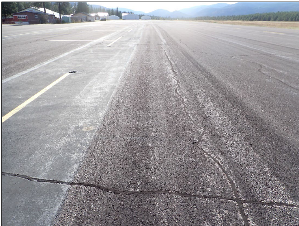
AP-03-07: L&T Cracking
