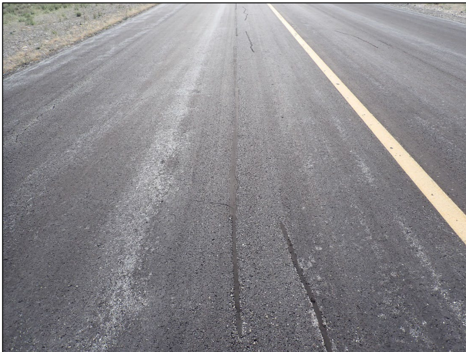
TW-05-04: L&T Cracking
