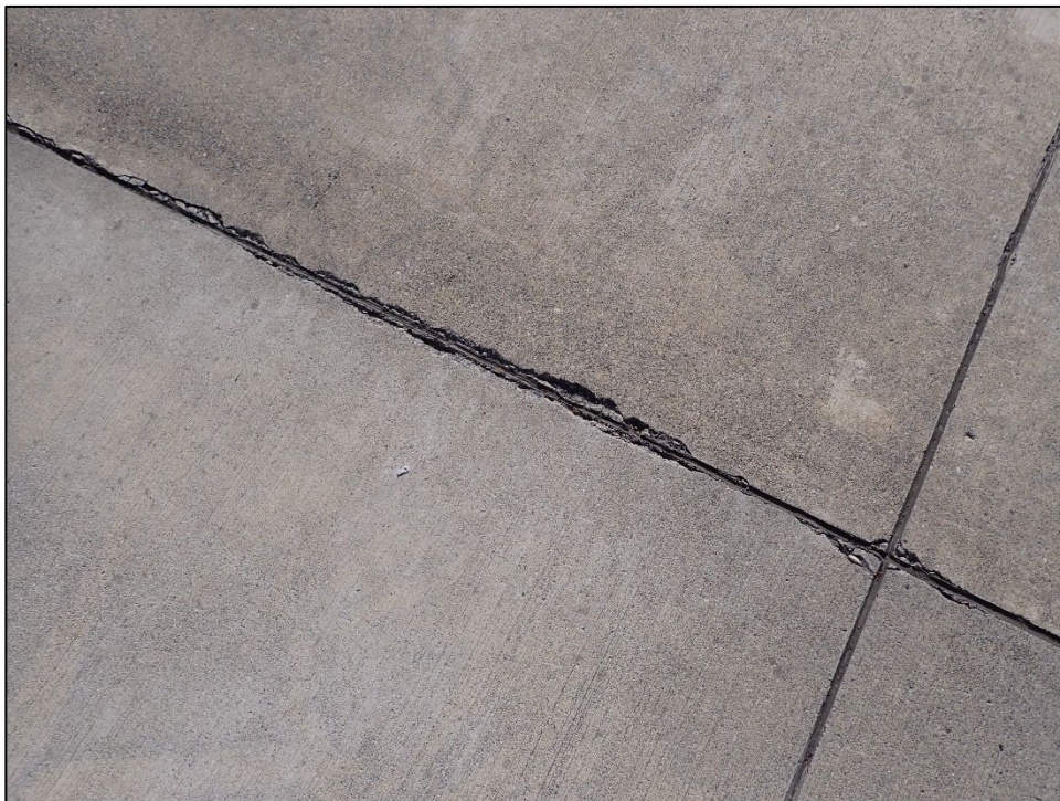
AP-06-02: Joint Spalling
