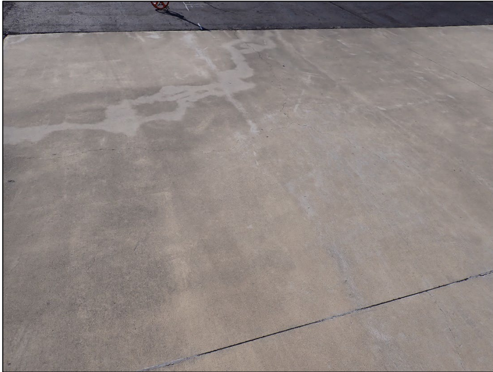
AP-04-01: Shattered Slab/Intersecting Cracks
