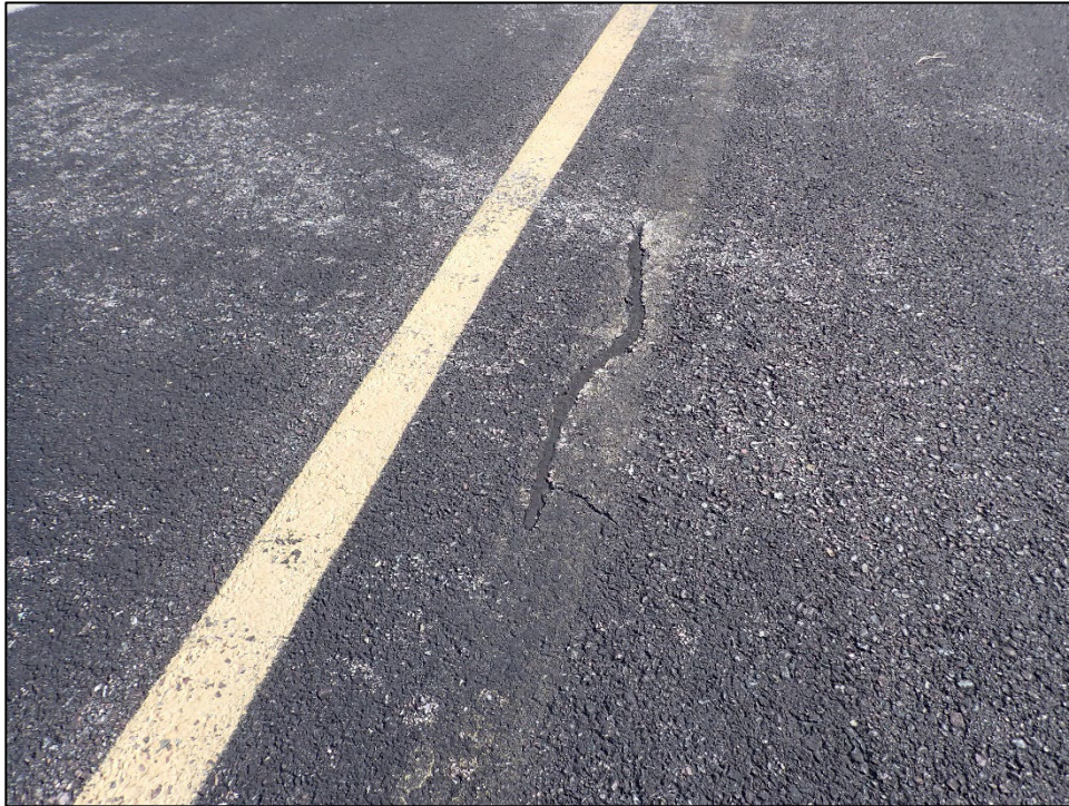
TW-03-02: L&T Cracking
